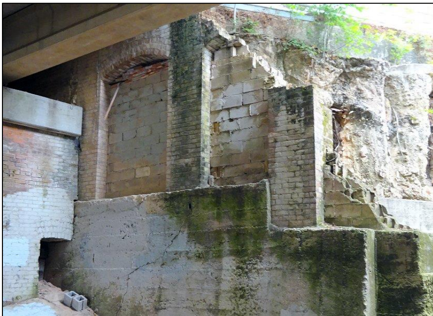
Figure 4: The right-hand wall of the Donnellan grave site contains two large masonry arches. The segmental style arches are similar in style to the small arch of the embankment wall. (Louis F. Aulbach)
